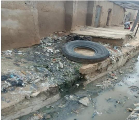
**Plate 5:** Bad Soakaway Releasing Wastewater at Unguwan Dacci
