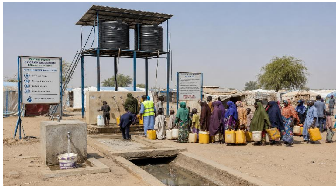
Figure 4. Water distribution point infrastructure in a Maiduguri-area IDP camp illustrating physical access conditions, queue management, and infrastructure quality typical of formal camp settings in north-eastern Nigeria.
